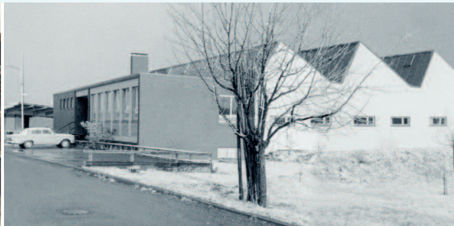
New building 1963 in Weinstadt-Grossheppach
